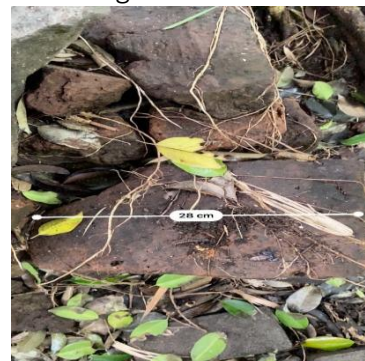
Figure 4. Brick Structure in Tambak Hamlet.
