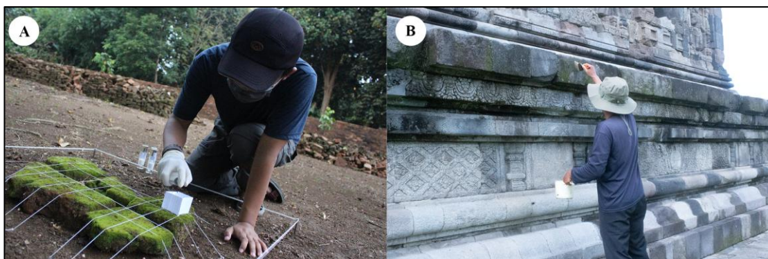
Figure 2. (A) Spraying Method in Muarojambi Temple Compound (Brick Temple) and (B) Brushing Method in Plaosan Temple Compound (Stone Temple).
